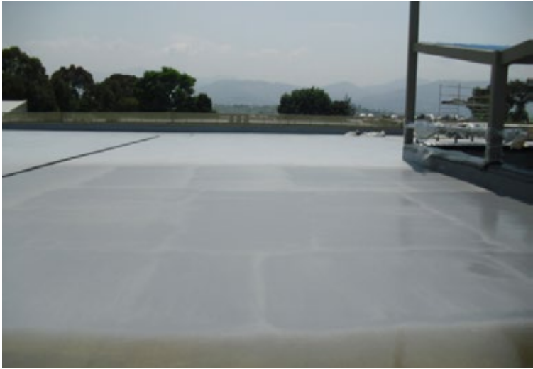
WATERPROOFING Projection of TECNOCOAT P-2049
