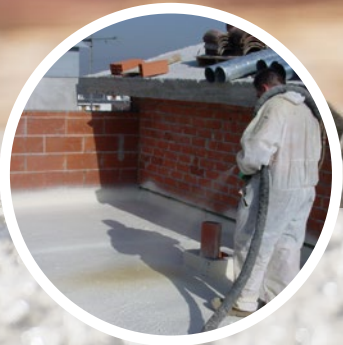
TECNOFOAM G-2060 FOAM DESIGNED FOR INSULATION OF INVERTED ROOFS
